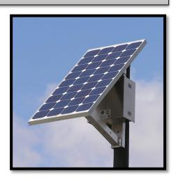
Solar panel assemblies are selected to charge the battery assembly to run the light fixture the needed run time operation of the project. The panel assembly is selected by the solar lighting specialist working on the project taking into consideration installation location, operation of the fixture and available sun hours.
