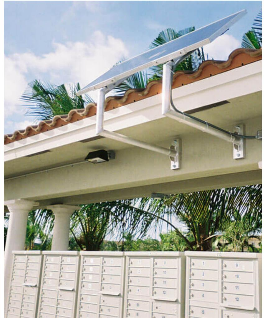
*High-powered LED fixtures can be used to provide optimum lighting levels for the application. SEPCO works with Hubbell Outdoor Lighting to provide different distribution patterns for every project maximizing the light output of each fixture. Since uniformity is key, creating a lighting layout for the application will provide the necessary information on the number and type of fixture required for the needed luminance for visibility.*
