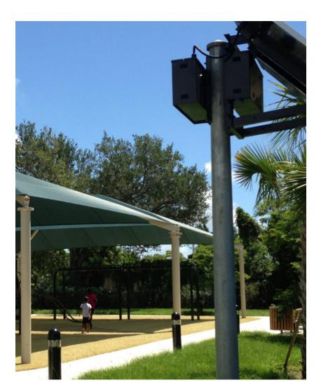
Each solar power assembly can operate one fixture or multiple fixtures depending on the requirements of the project. For example, a sign may require anywhere from two to six fixtures, all powered by a single power assembly. Same thing can be done with pathways using bollard fixtures. Most overhead systems are powering a single or double fixture arrangement.
