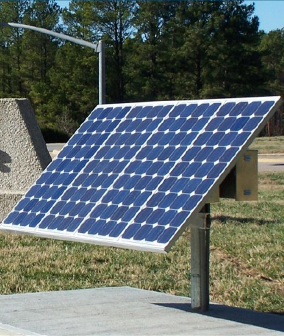
*Part 5 of the solar lighting design guide is about determining the power assembly. Now that you know what area of coverage you are requiring by determining the lumen requirements for the project, as well as the required operation profile, it is time to determine what size solar power assembly will be required. This is determined by a simple calculation after some additional information is gathered.*
